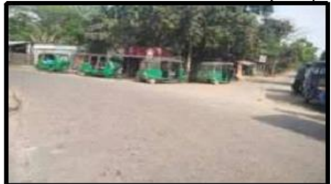
Fig. 5: No Channelization at the Intersection, no Marking (Road # 1)
