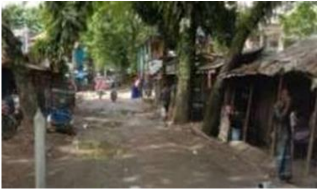
Fig. 6: Damage Road Surface (Road # 5)
