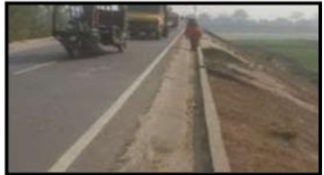
Fig. 11: Open Surface Drain, Steep Fill Slope, no Barriers (Road # 4)
