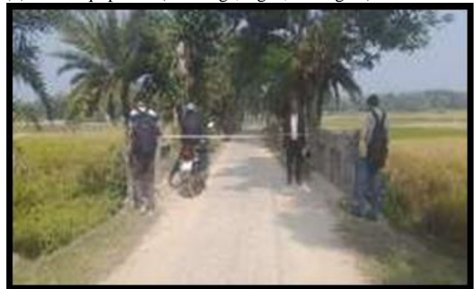
Fig. 4: Narrow Road and Shoulders Occupied by Trees (Road # 8)
