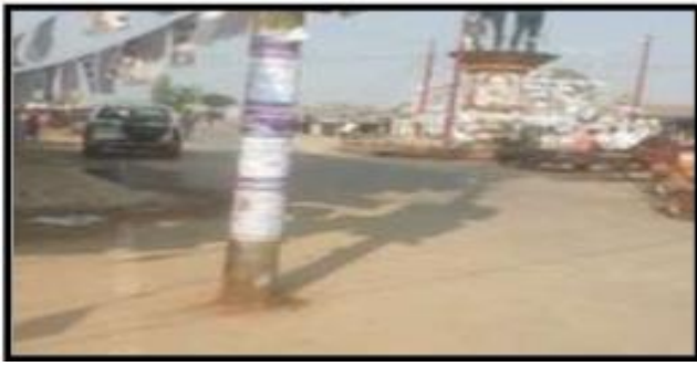
Fig. 14: Utility Pole on the Carriageway (Road # 4)
